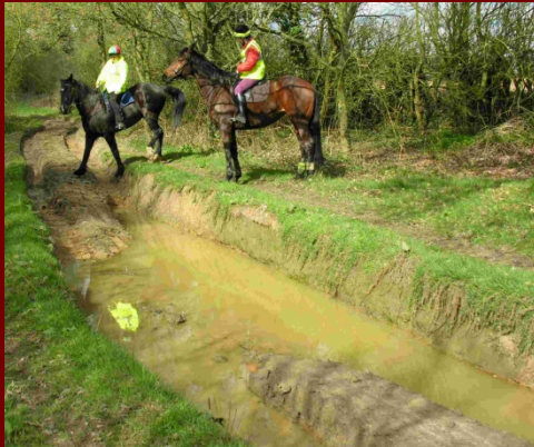
Poorly maintained surfaces
