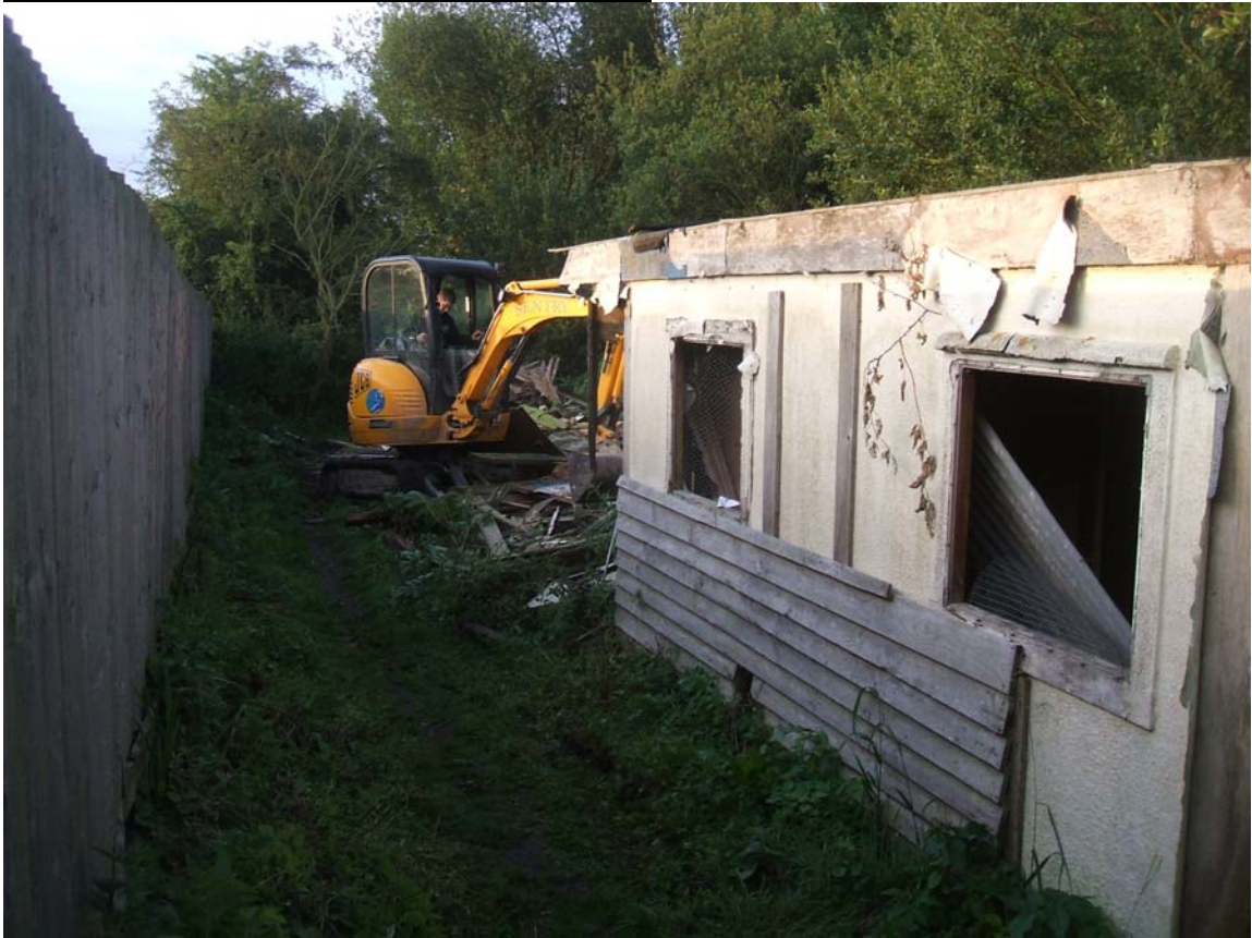
Tring Rural FP043 Enforcement Works.
