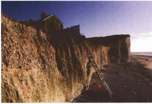
Coastal erosion at Birling Gap, East Sussex
